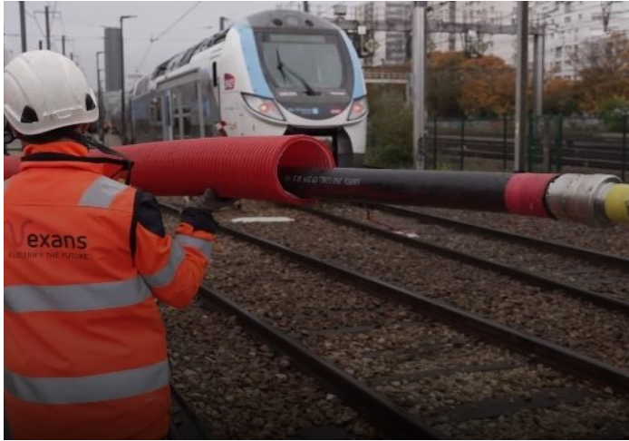
SUPERRAIL SNCF PROJECT Paris, France
