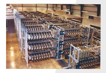
Two ± 160 MVA VSCs at AEP Inez Substation. One of the VSCs can be operated in SSSC mode.
